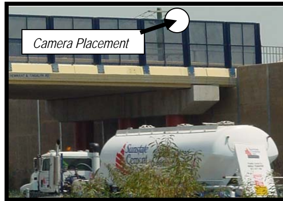
Figure 1 Hemmant & Tingalpa Road overpass, Port of Brisbane Motorway
