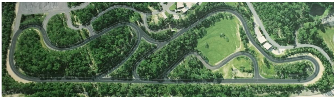
Figure 5-5: Aerial view of the closed road circuit
