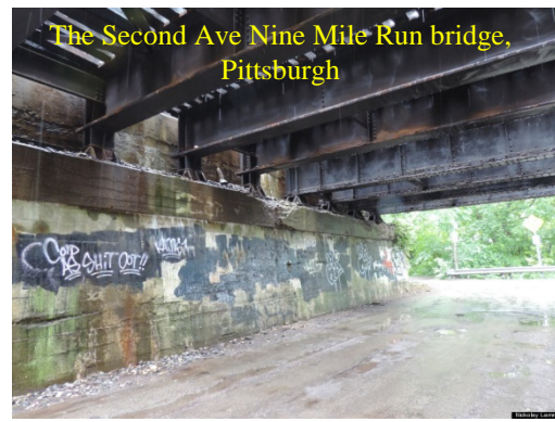
Figure 1.1: Deteriorated steel structural members
