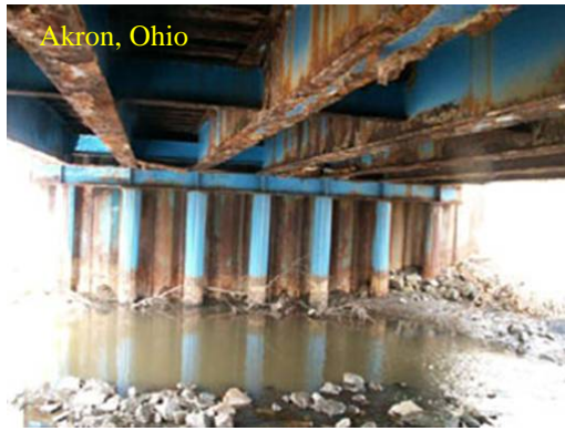
Figure 1.1: Deteriorated steel structural members
