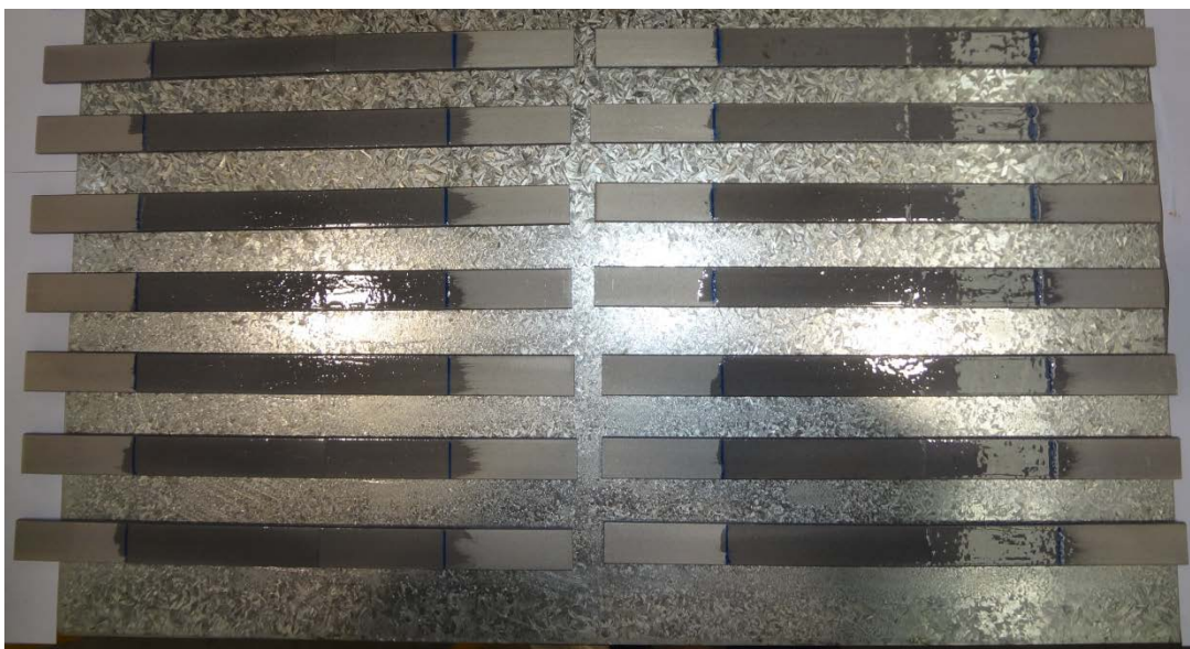
Figure A2: Application of primer coat
