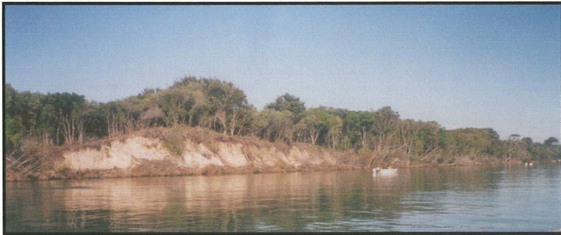
Figure 39. Site MDE5. An example of erosion on the mainland side of the sand spit, adjacent to Pumicestone Passage. The scarp is approximately 4 m high, with fallen vegetation at the base. Six monitoring sites were established at this site (sites MS1 – MS6).
