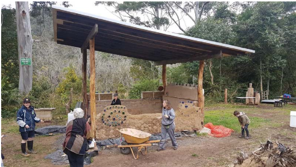
Figure 23: NEV members building an outdoor kitchen.
