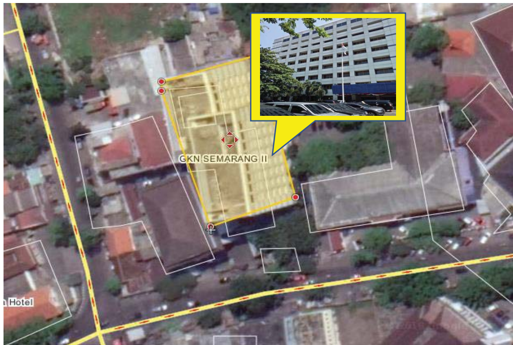
Figure 6.2 Satellite view of State Finance Building II Semarang
