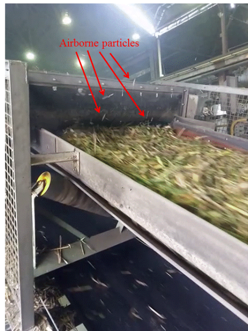
Figure 1. Inlet to the Tully shredder operating prior to the installation of the added windage plate showing particles that were made airborne by windage near the curtain.
