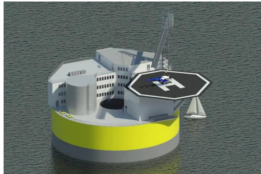
Fig. 5b Floating nuclear power plant
