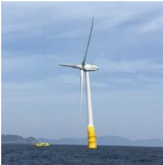
Fig. 1a Floating spar wind turbine, Goto Island
