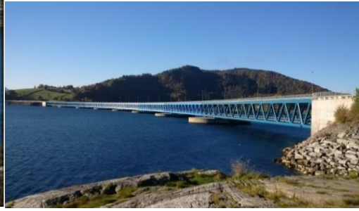
Fig. 25d Bergsoysund Bridge
