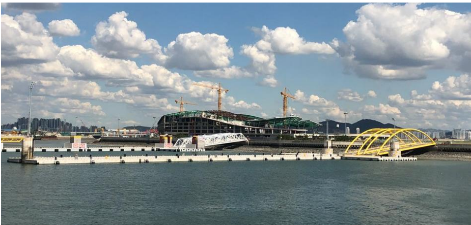
Fig. 26 Floating piers in Incheon Golden harbour (photo courtesy of Kwanghoe Jung)
