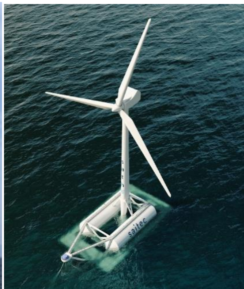
Fig. 1b Saitec wind turbine on concrete pontoon off the coast of Spain
