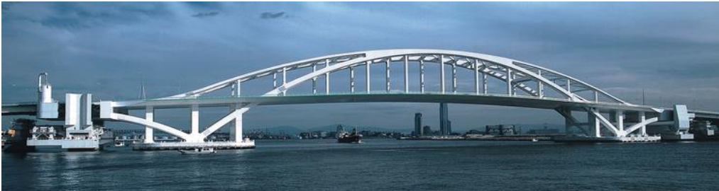
Fig. 25e Yumemai Floating Steel Arch Bridge in Osaka
