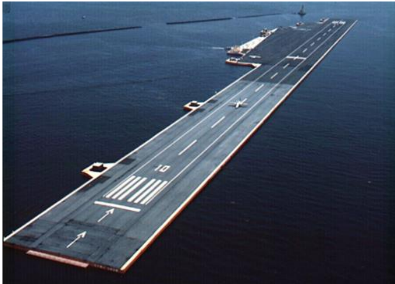
Fig. 27 Mega-Float – a 1 km long floating airplane runway test model in Tokyo Bay (photo courtesy of M. Fujikubo)
