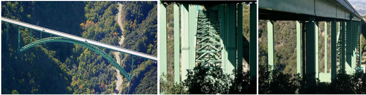
Figure 7: Cold Spring Canyon Bridge
