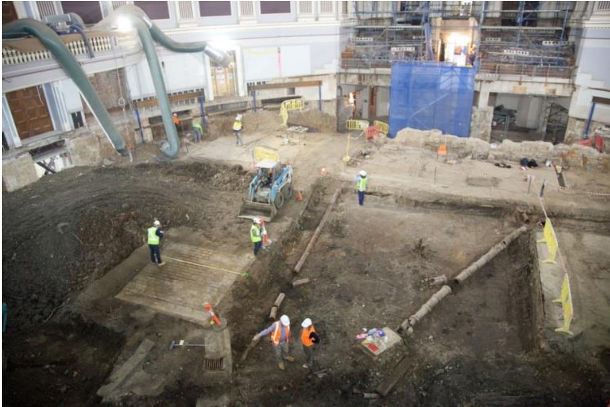
Figure 11: Cobblestone drain, pipes and paving (Brisbane City Council, 2013)
