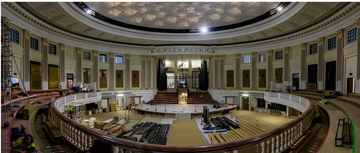
Figure 7: Finalising work in the Auditorium in November of 2012 (Brisbane City Council, 2012)
