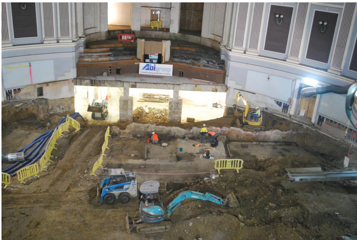
Figure 10: Excavation work under the auditorium floor (Brisbane City Council, 2013)
