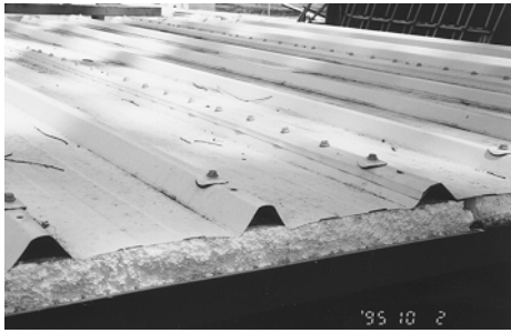
Seam fasteners at closer spacing
