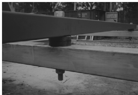
(c). Purlin to Rafter Joint
