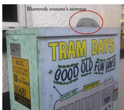
Figure 3-1: A photograph of a BMS equipped signal controlled in Brisbane with a shark fin shaped BMS antenna on the top
